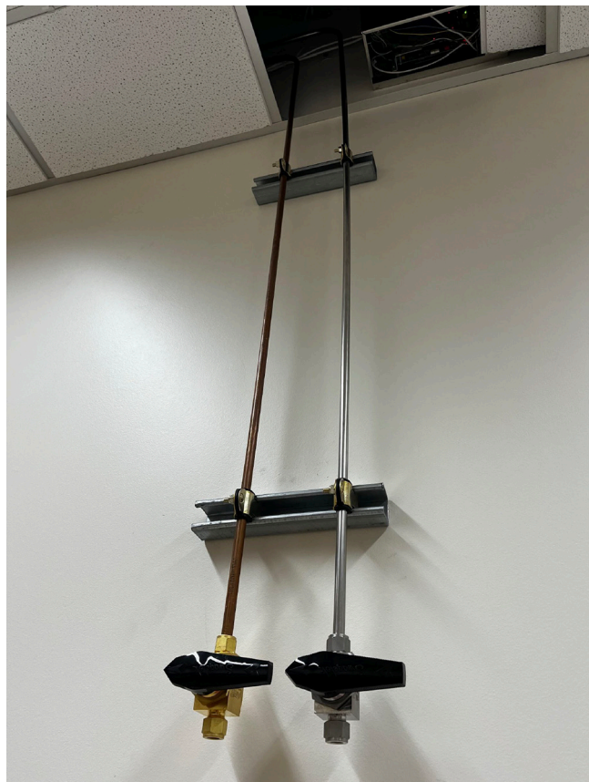
Figure 2: Compressed Air (left) and House Nitrogen Gas Lines Ran in Lab 238. We installed six of these valves and their pipework under Paul's supervision.
